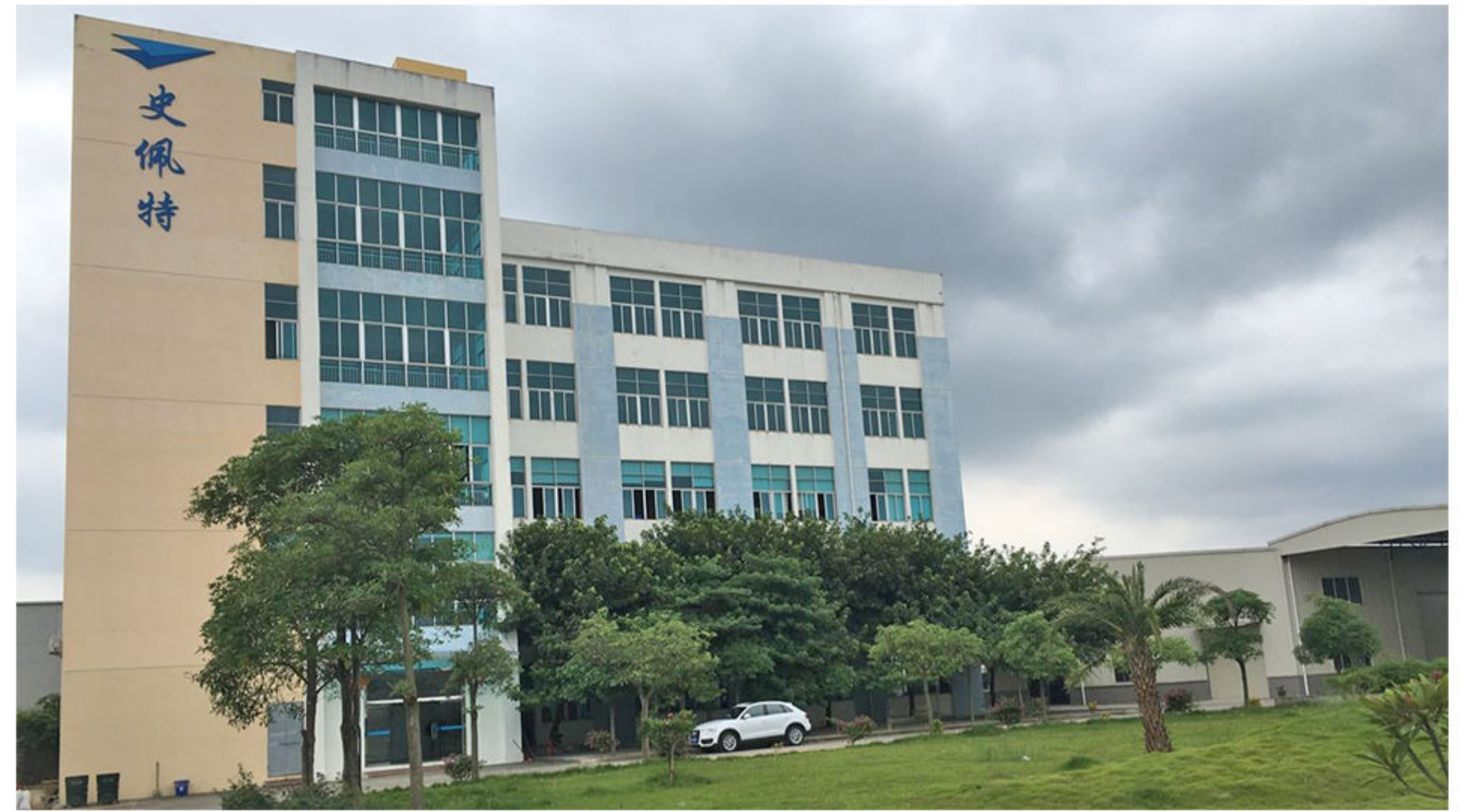
Sharp Point Component Plant, China
